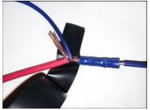
**Electrical Taping Bare Wires**
